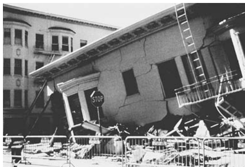
Figure 3.3 This building in San Francisco was wrecked when its lower floors gave way during the 1989 Loma Prieta earthquake.
